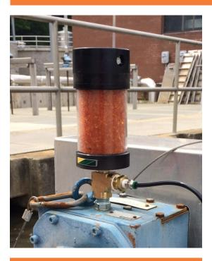
The Watchdog EX Breather is used to protect the integrity of in-service lubricants by mitigating contaminants from entering the system while allowing the system to breathe when required. Contaminants are removed via a bed of desiccant and 2 micron filters (desiccant never comes in contact with lubricant).
